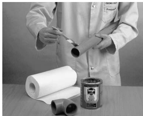
Applying the cement
