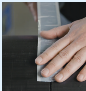
Seal the jointing face between the fitting and pipe with sealing tape and shrink the shrink sleeves.
