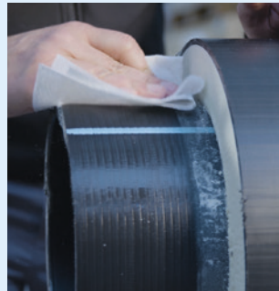
Peel the ends of the pipe and fitting type B and clean the fusion zones of the fitting and pipe using a clean cloth.
