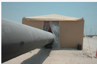
Protecting the welding zone using a tent
